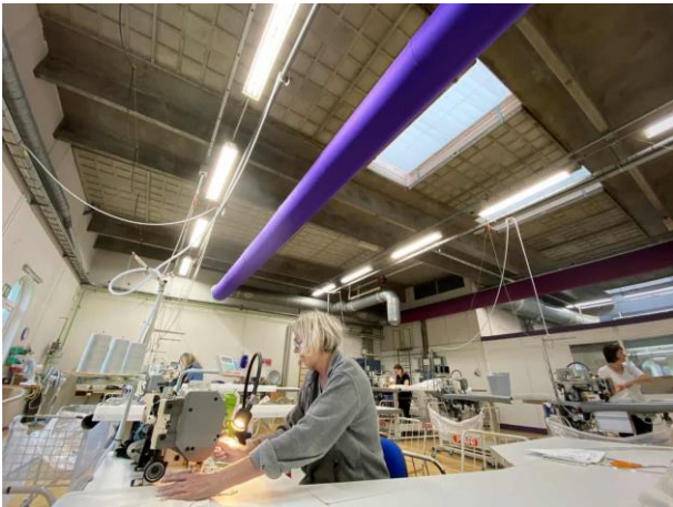
KE Fibertec's ventilation system consists of woven special fabrics that are sewn into textile ducts such as this purple ventilation duct under the ceiling. Photo: Søren Dippel
