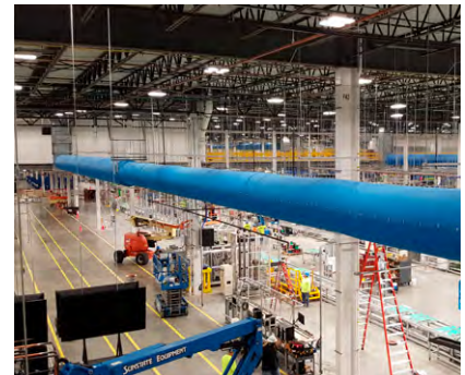
Daikin Texas Technology Park, USA
