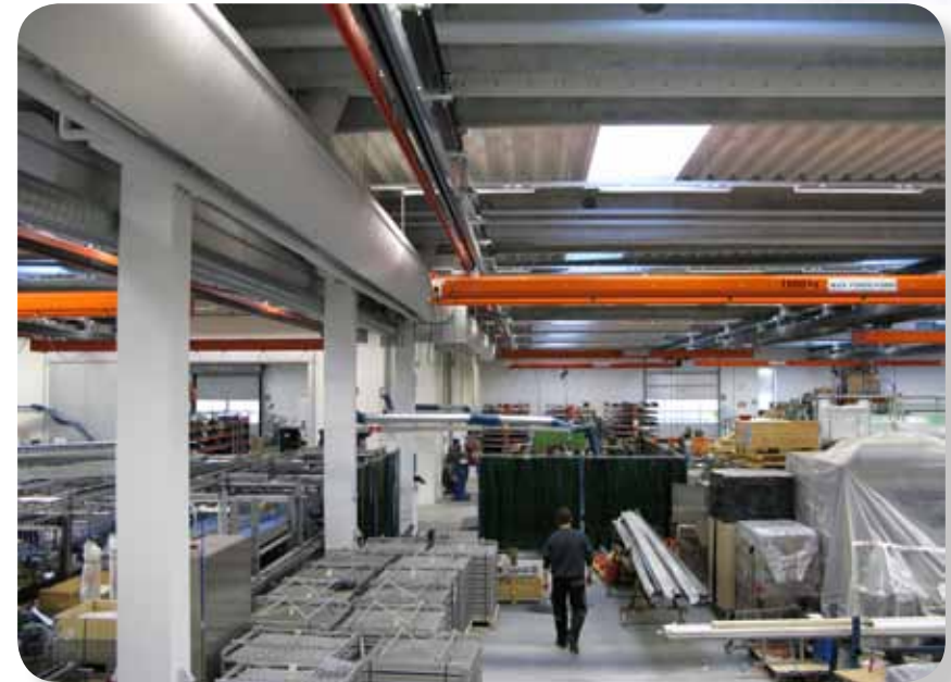
Round KE DireJet textile ducts
