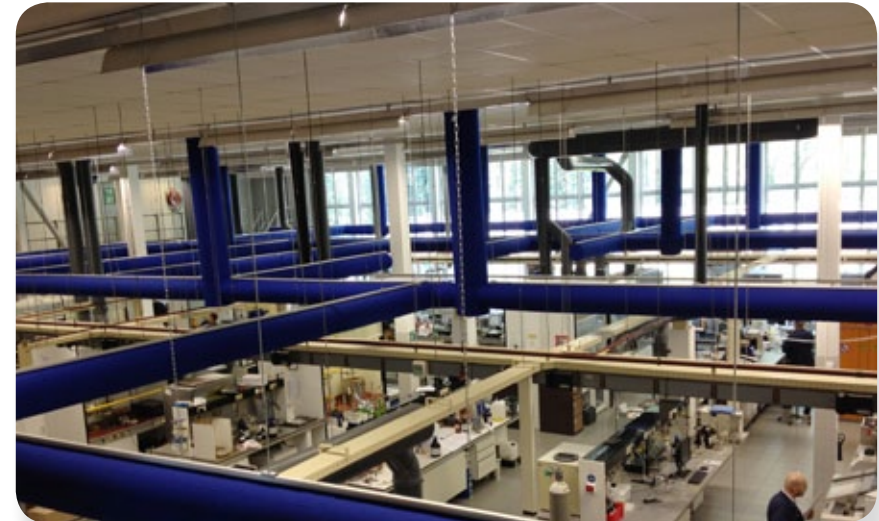
KE Hybrid (Low Inject) Ø400 and Ø300 textile ducts
