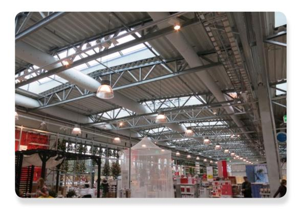
The system is manufactured in sections of each 5 metres that are connected by means of zippers. The sections are suspended in the ceiling using double rows of aluminium rails. Naturally, the textile material is fire retardant.
