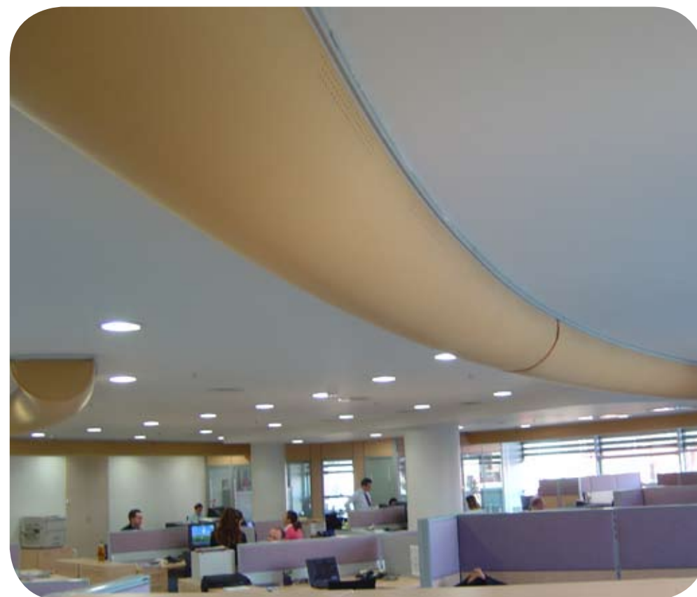
KE-Interior System with curved ducts and rails
