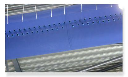
Waste heat is recovered (> 80%) for heating of the halls. The recovered heat is efficiently distributed to the halls by means of DireJet systems thus rendering the KE systems very suitable both for make-up and process air as well as for heating.
