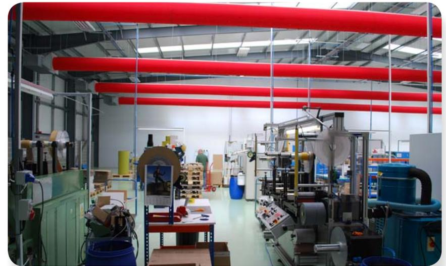
*KE DireJet textile ducts with Ø18mm nozzles*
