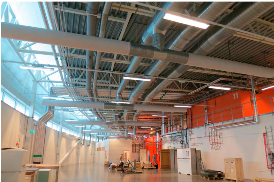
Ring structure in main building
