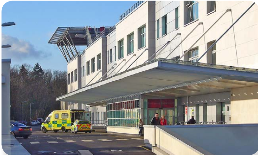
Broomfield Hospital, Chelmsford, UK
