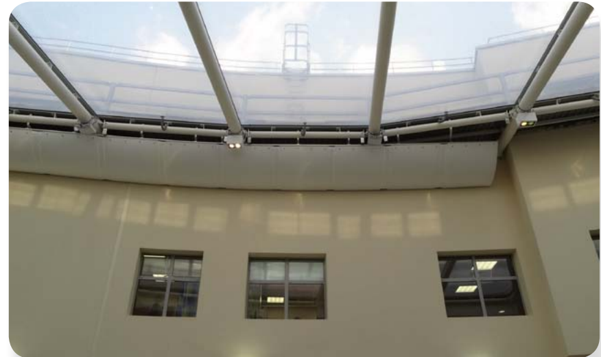
KE DireJet textile ducts with 24mm nozzles
