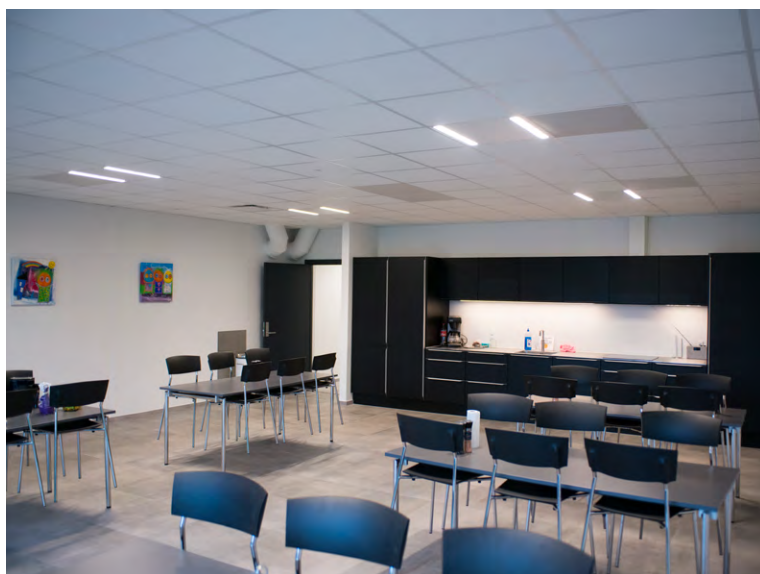
FBS loftpaneler i administrationsbygning
